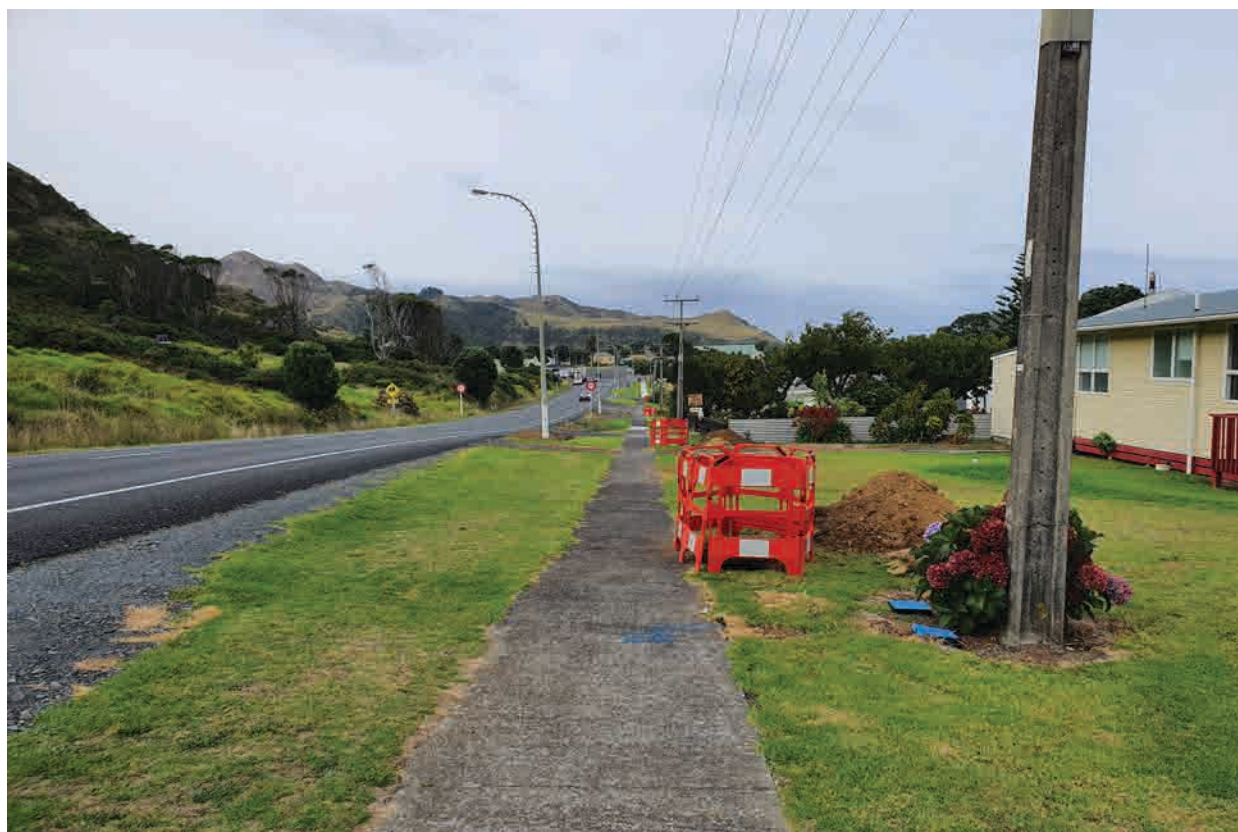
Figure 4. View south down SH3 of insertion holes inspected prior to drilling.
